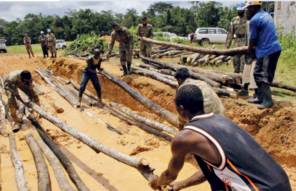
Pakistani troops and Liberian villagers repair a flooded road on the outskirts of Voinjama, Lofa County.
